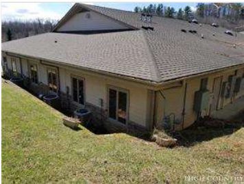
East Side and Back of Building
